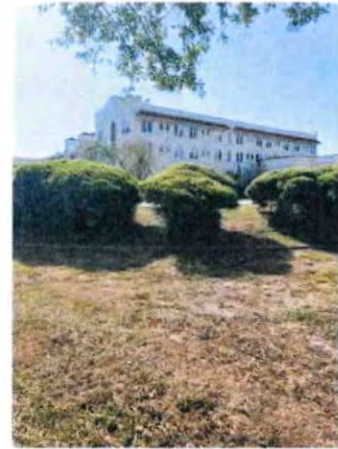
Photograph #5D - Facing Southeast
