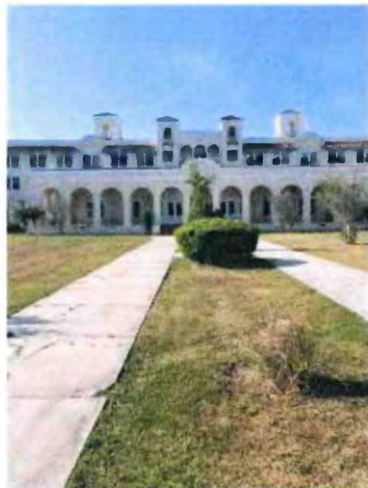
Photograph #4C - Facing South
