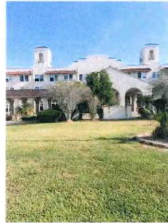
Photograph #1B - Facing North
