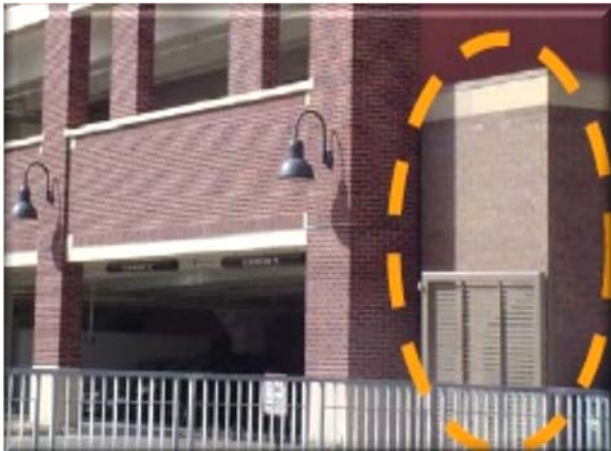
Equipment is shielded from the right-of-way with a masonry structure attached to a parking garage.
