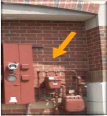
Utility equipment is painted to blend with the building.
