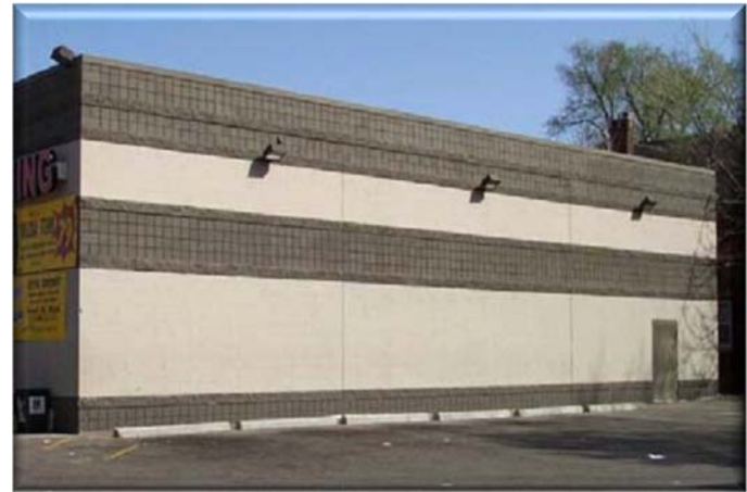
Blank wall facing the parking area which is visible from the street. The blank wall is painted plain and scored concrete block with only an emergency exit at the end of building.
