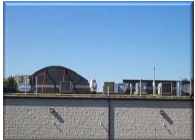
Unscreened rooftop mechanical equipment.
