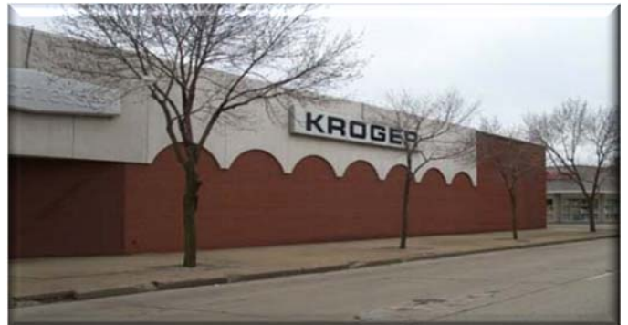
Store has attempted to enhance the blank wall by applying arches on the brick surface in a different material and color and placement of sign. Unfortunately, this side is missing entryways, storefront and display windows.
