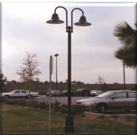
The downward facing light illuminates the parking lot without causing glare.
